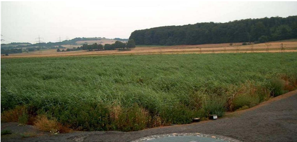
Fig. 14. Advanced wastewater and sludge treatment using artificial wetlands in Fronhausen, Germany. [15]
