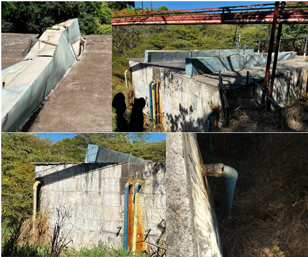
Fig. 13. Status of Barichara wastewater treatment plant. [8]
