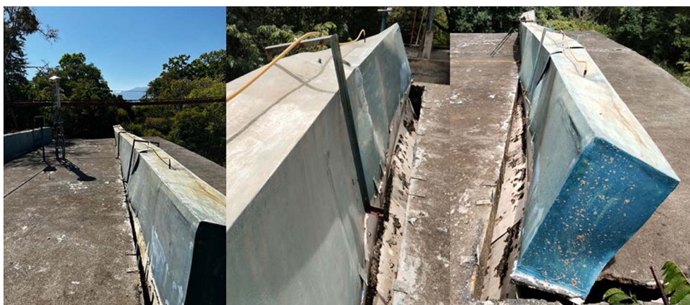
Fig. 11. State of methane gas pipelines. [8]
