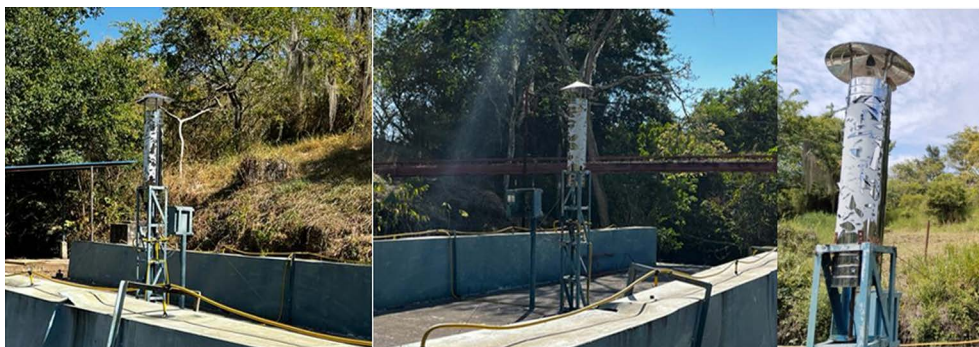
Fig. 12. Methane gas burner. [8]
