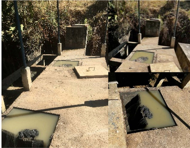
Fig. 7. Status of screening screens, Barichara WWTP. [8]
