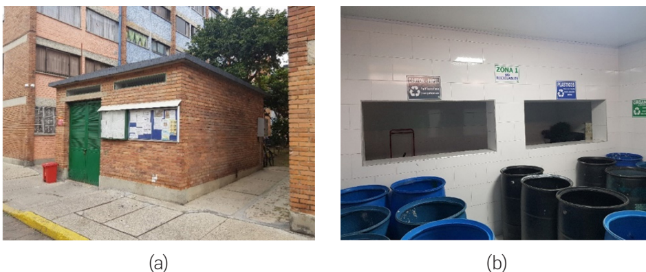
Figure 3. Temporary solid waste storage room, (a) exterior, (b) interior. Source: Authors
